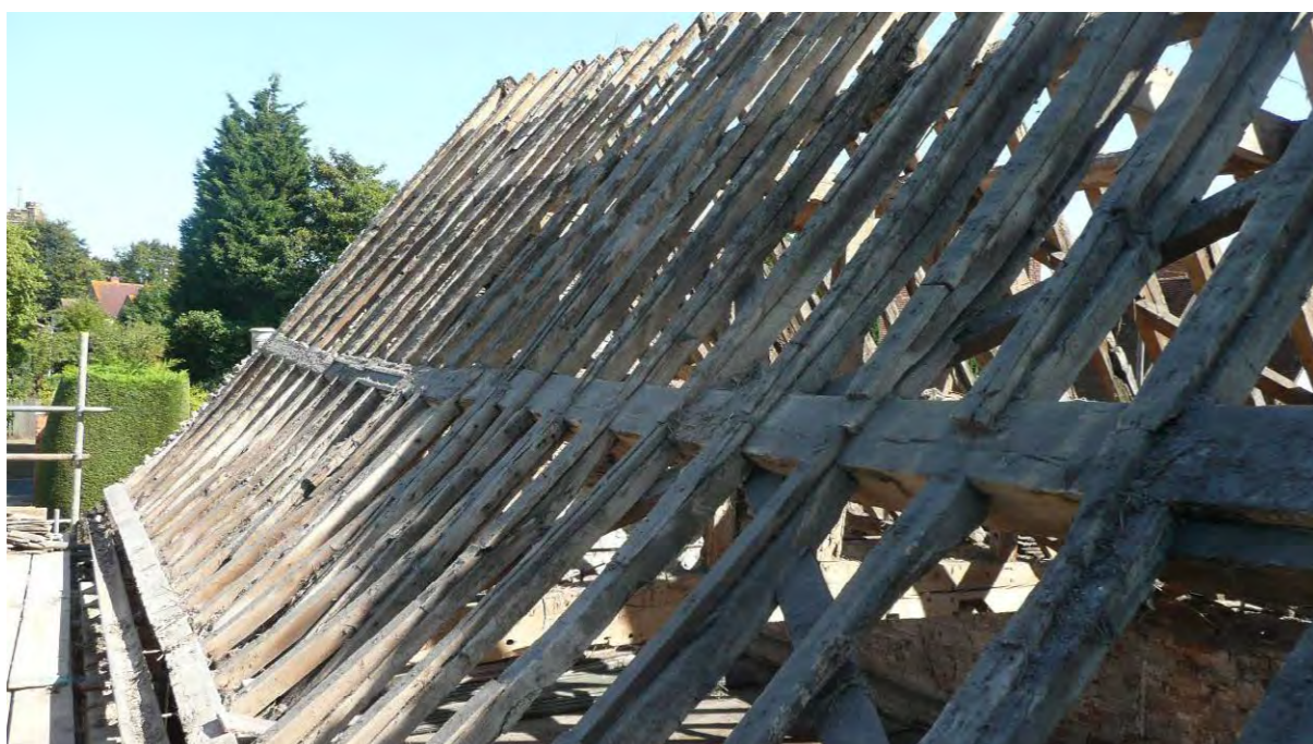
Figure 21: (top) Interior of former Town Hall, Toddington Figure 22: (bottom) Re-roofing of the stables at Harlington manor
