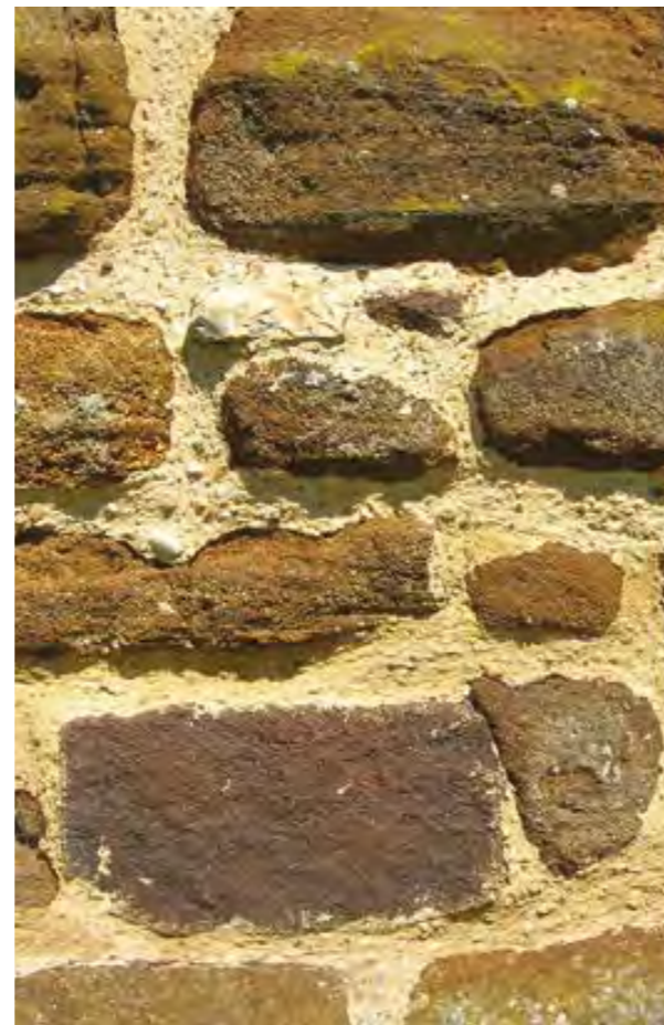
Figure 71: (bottom right) Ironstone repointed using lime mortar and a sharp gritty sand providing a traditional finish which will preserve the integrity of the historic stonework Figure 72: (left) Barn at Barton le Clay showing different depths of weatherboarding Figure 73: (top right) Example of good practice timber repair – sections of timber being spliced in retaining as much of the historic fabric as possible
