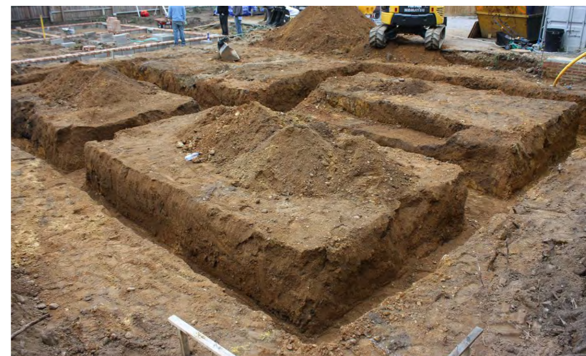
Figure 59: Flitwick construction impact
