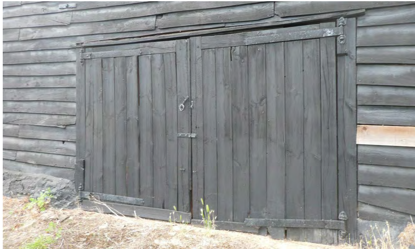
Figure 24: New openings should be kept to a minimum and cart openings and doors such as those at Crawley Hall Barns, Husborne Crawley should be retained as part of a conversion scheme.
