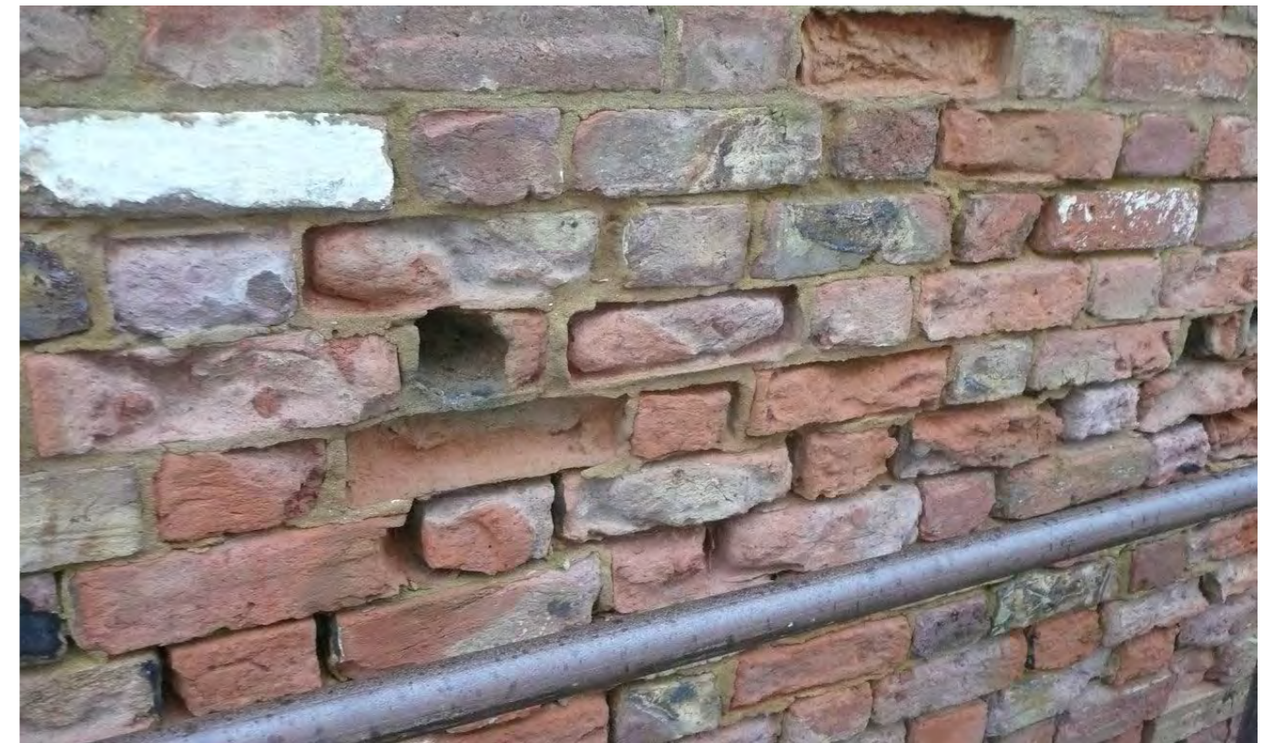
Figure 74: (top) West Front of St Peters Figure 75: (bottom) The damaging effects of cement painting
