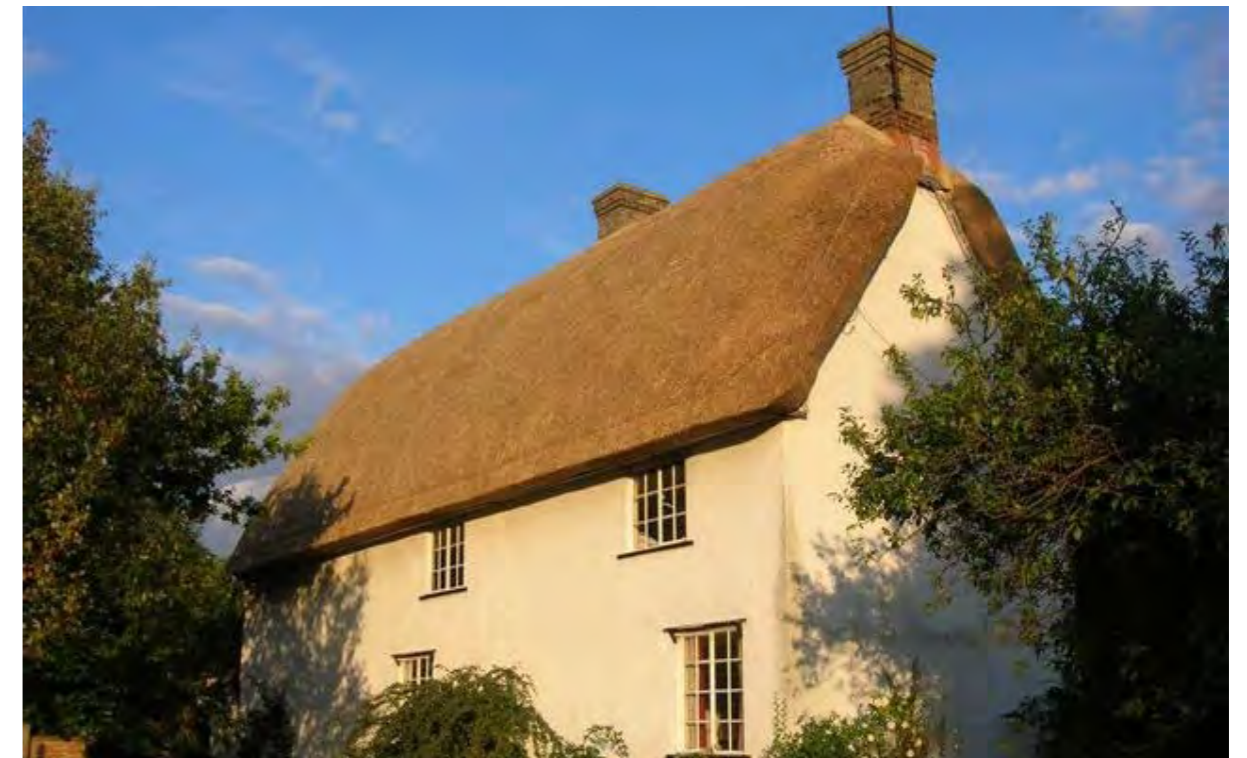
Figure 64: Long throw thatched cottage, Wrestlingworth - application of vernacular materials contribute to local distinctiveness
