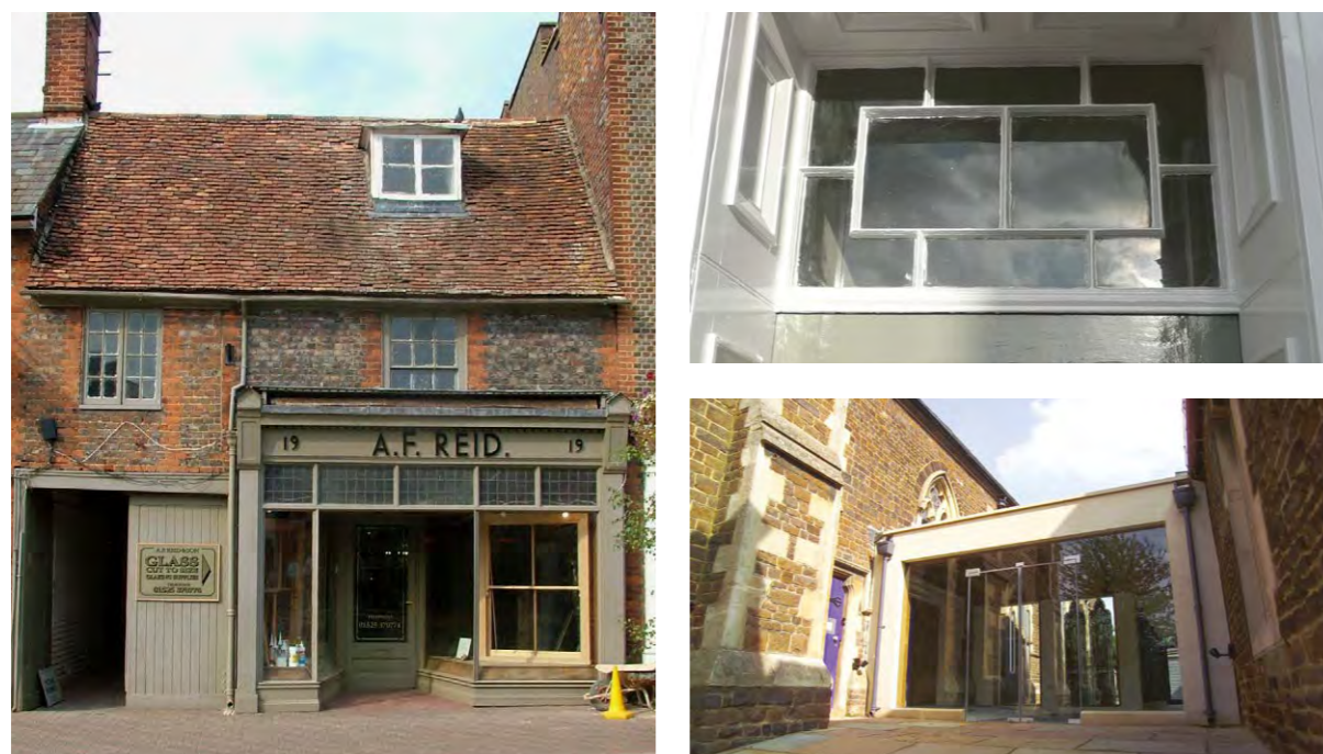
Figure 37: (left) Very good example of a traditional shopfront – Leighton Buzzard Figure 38: (top right) Fanlight, Linslade. A feature which contributes to historic character Figure 39: (bottom right) Sympathetic contemporary addition creating a foyer to a Victorian church, Linslade
