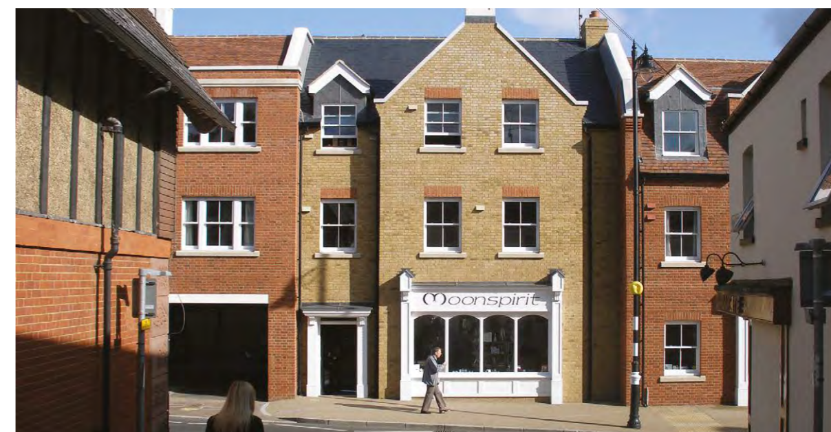
Figure 40: Recent development incorporating a shopfront elevation designed as an integral part of the street scene and to terminate the view from a side street.
